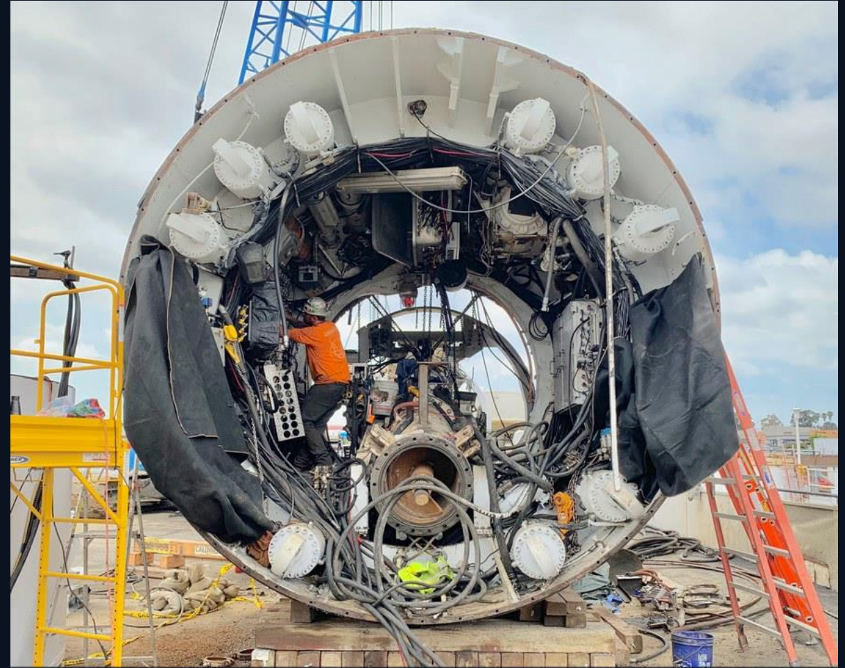
Boring Company TBM
